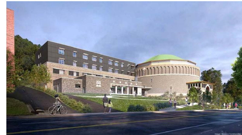
North Negley Residence (13 PBV, 35 Other Affordable units) Under Construction
