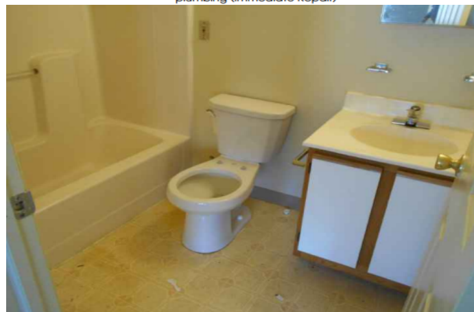
59: Replacement of dwelling unit flooring and vanity (Immediate Repair)
