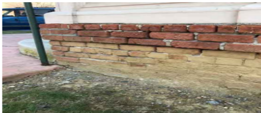
48 - REPOINTING OF BRICK
