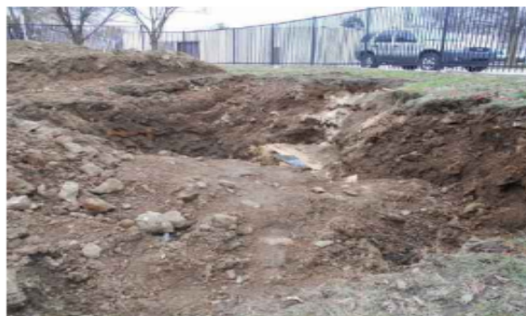
10. Domestic water supply repair (Critical
