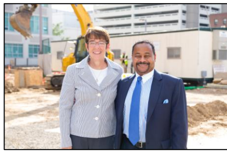
Brian Hudson, PHFA executive director, and Sister Mary Scullion, Project HOME, were present during the groundbreaking ceremony of the 810 Arch Street project, Philadelphia, in mid-September. The nine-story mixed-use development will provide retail space and 94 housing units for formerly homeless and low-income men and women. Photo courtesy of Jay Gorodetzer.
